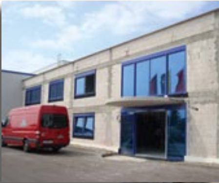
In progress: the new DTS office building and showroom
