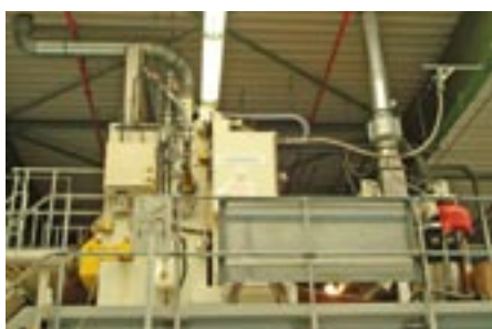
Electronic beam curing unit
