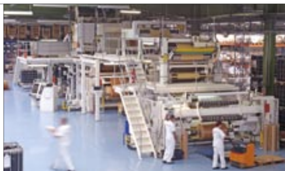
The complete electron beam curing line which costs more than EUR10 million each
